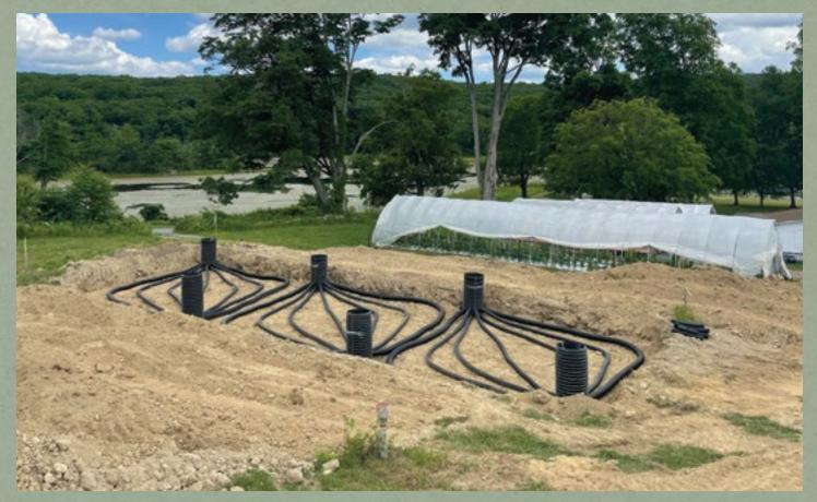
Climate Battery Greenhouse while being constructed—the underground network of pipes distributes the warm air captured above, Credit: Glynwooc
